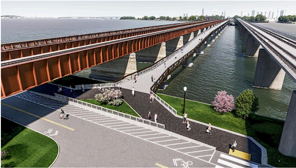
Long Bridge project across Potomac River includes a separate bike/pedestrian bridge
